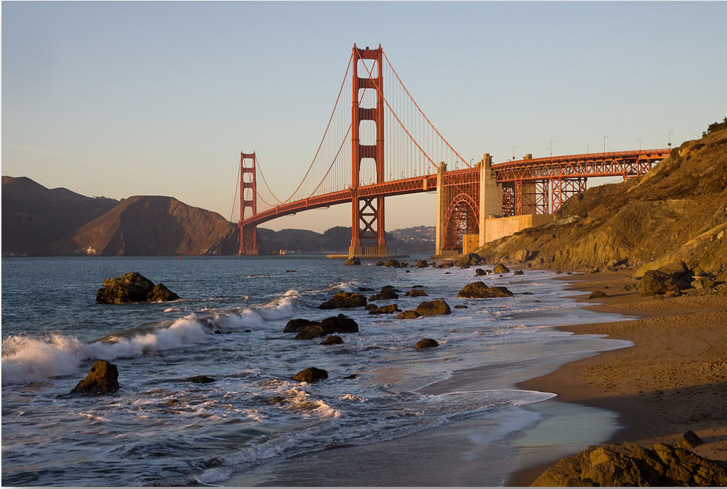
Golden Gate Bridge
